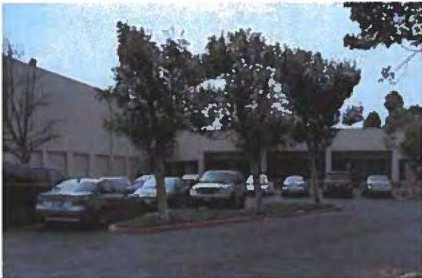
View of the Robinson Pharma office from the North.
