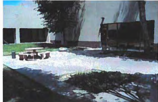
General view of the courtyard area on the south side of the Robinson Pharma space.
