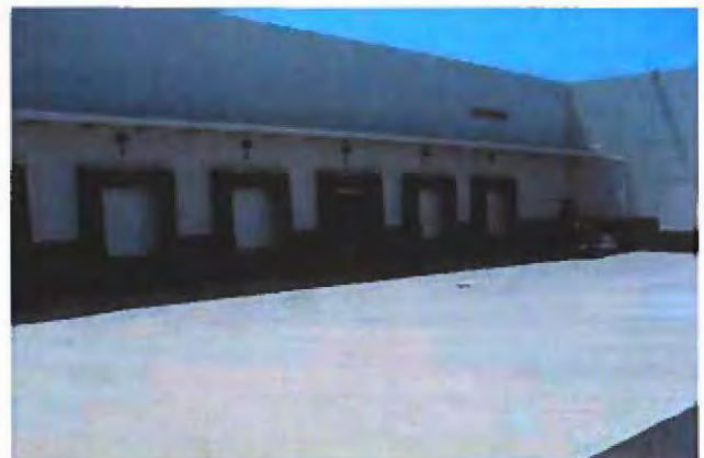
View at the TY North America loading dock area.
