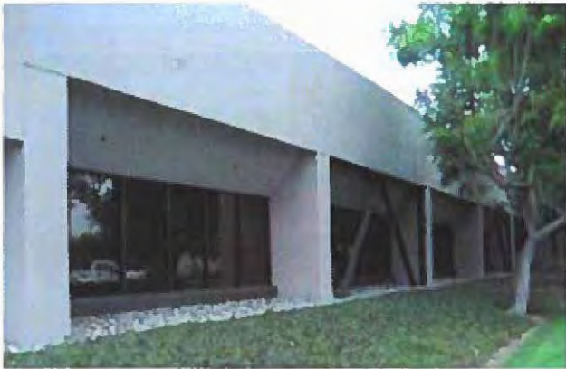
View of the Robinson Pharma office area facade.
