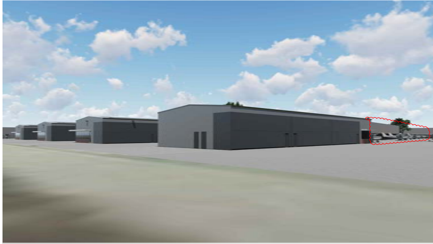
VIEW SOUTHWEST FROM AIRSIDE 1
