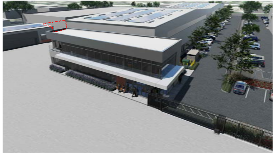
AERIAL VIEW WEST OF FBO AIRSIDE 4
