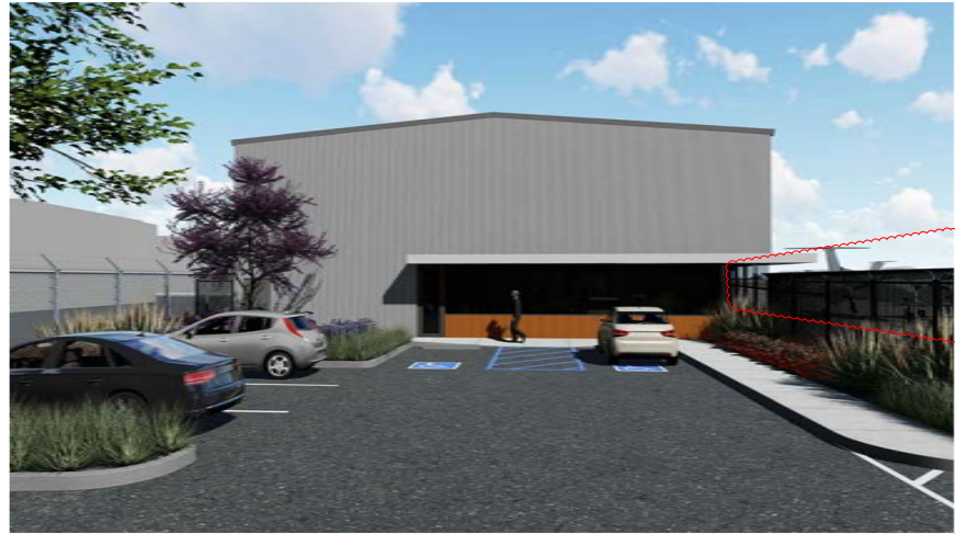
VIEW WEST FROM AIRSIDE 4
